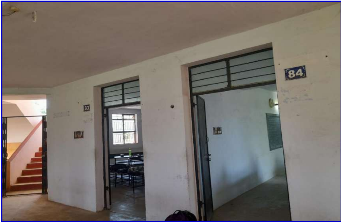
INFORMATION TECHNOLOGY UG CLASSROOMS
